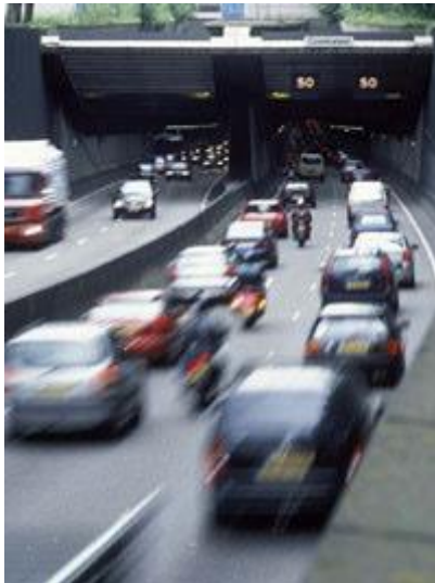
Figure Existing Coen tunnel
